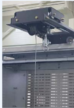
Hoist mounted on switchgear
