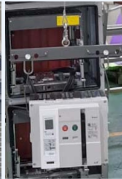
Hoist mounted on switchgear
