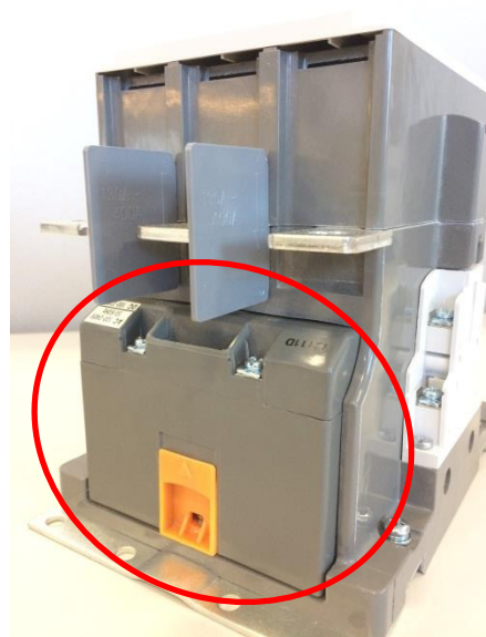
2. Locate the contactor coil.
