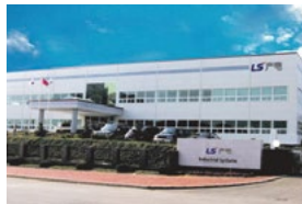
Dalian Factory (China) MV/LV Switchgear, and MV Contactor
