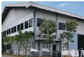
Tangerang Factory (Indonesia) Pad TR, Distribution Oil TR, and Distribution Panel
